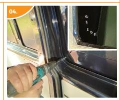
From the inside, drill the 5 'marker holes' in each corner where glass is being fitted.
