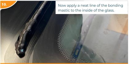
On opening windows, put a thinner amount on the plastic drains, so the mastic does not bulge out and block the drain holes.
