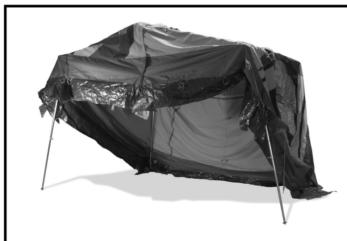
2. Lay awning material over the top of the frame
