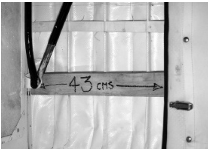
16. Chock your roof up with 43cm long pieces of wood
