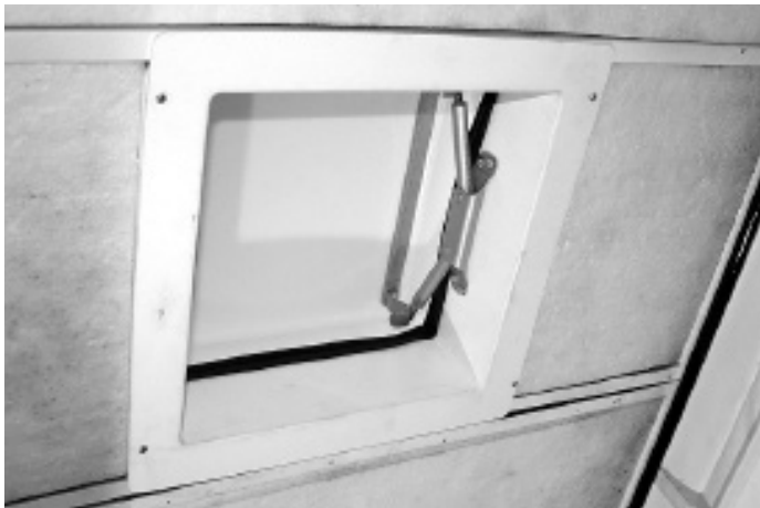
14. Bolt up the funnel and install the skylight mechanism
