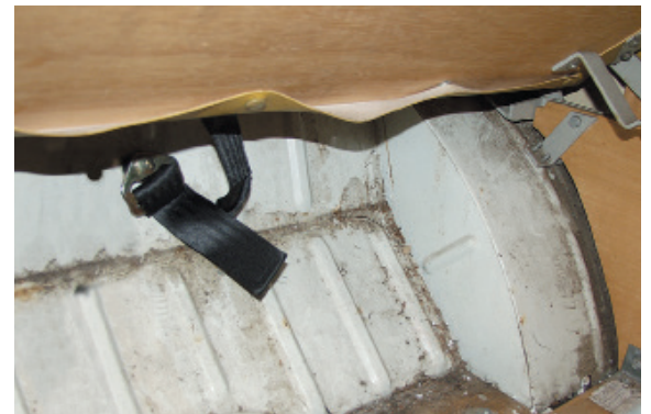
3. Non standard mounting in rear bulkhead
