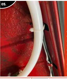
Make sure you only use plastic cable ties, as they are designed to melt in the case of a fire and allow the hose to drop into the fire area and speed up the process of the hose rupturing.
