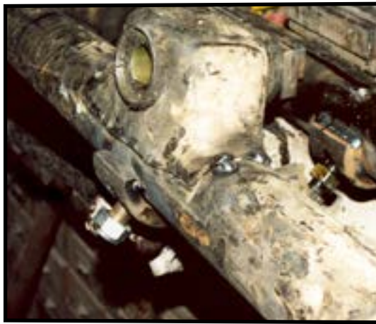
10. Weld the knuckle back on
