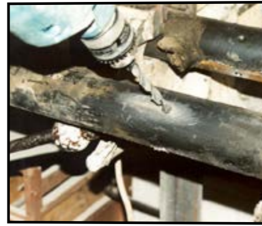
4. Carefully drill out the spotwelds
