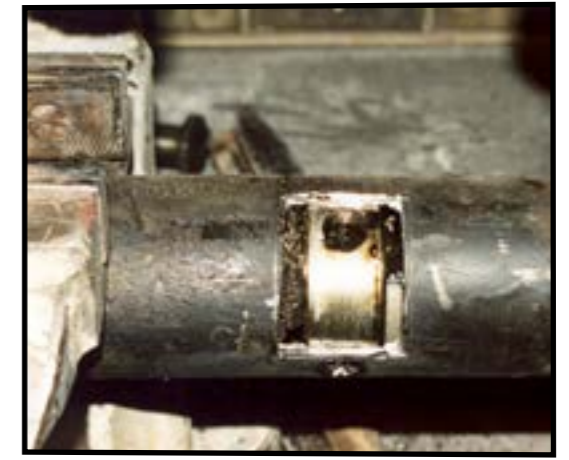
8. The cut beam with the centre exposed
