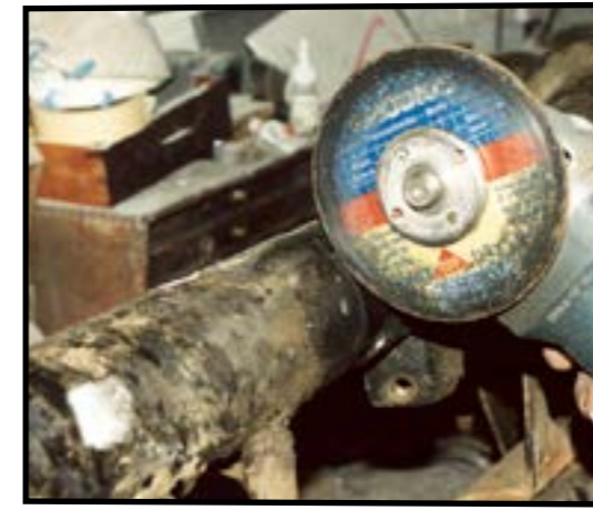
7. Carefully cut the beam
