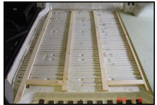
B. Bond wooden battens to the floor.
