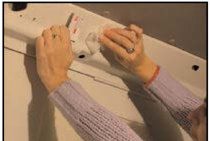
F. Wipe cant rails with surface cleaning tissues provided.
